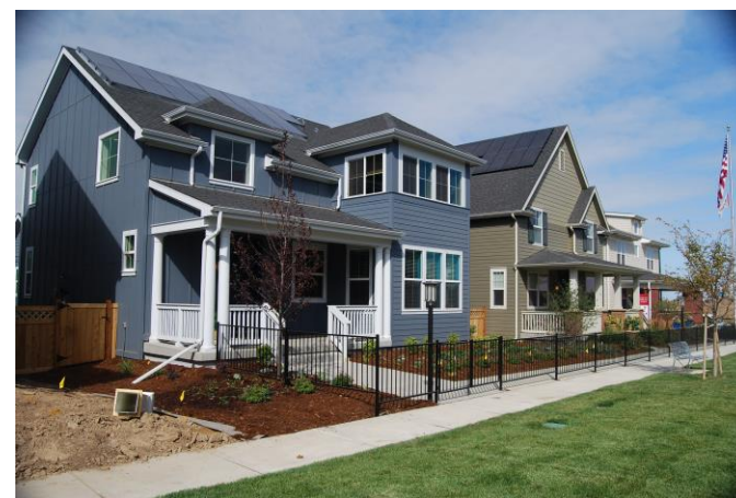
New Town Builders Zero Energy Home
