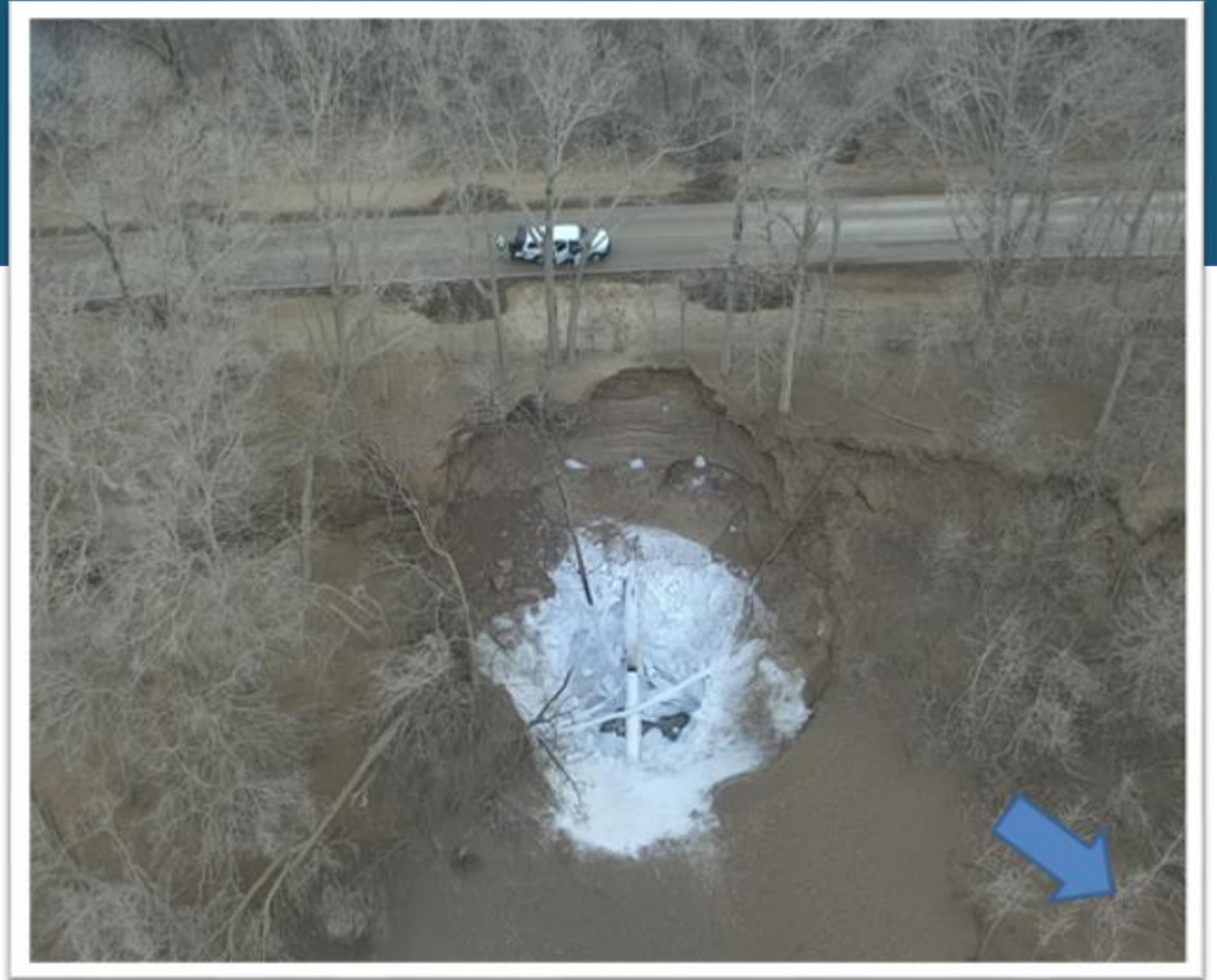
Aerial photo of pipeline rupture, Satartia, MS. From PHMSA's Failure Investigation Report – Denbury Gulf Coast Pipeline.
