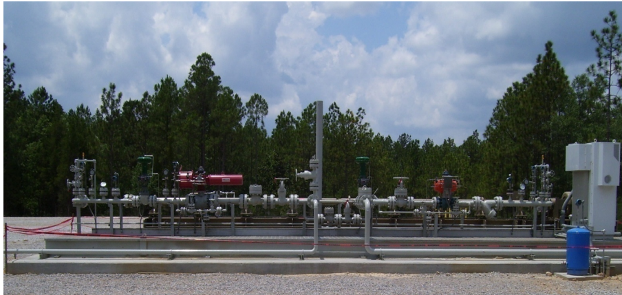
Horizontal CO 2 Booster Pump @ D-9-7 #2 Wellsite
