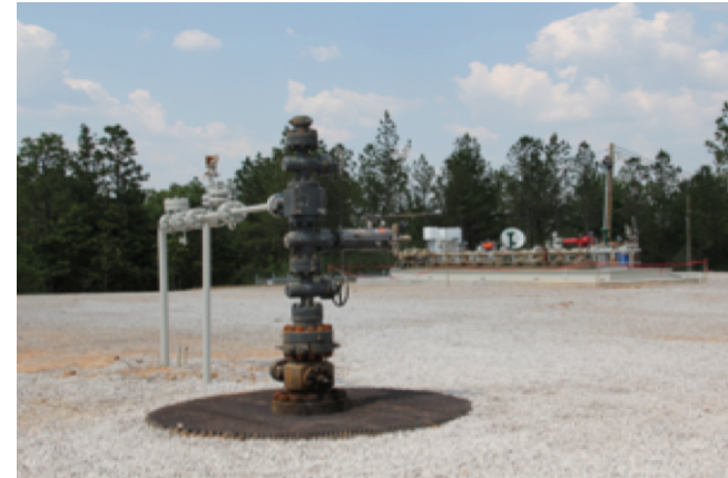
D-9-7 #2 Injection Wellhead
