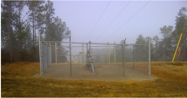
Mainline valve station along pipeline
