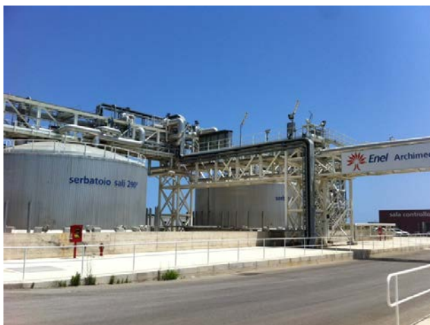
Figure 7. Enel's Archimede Concentrating Solar Plant stores thermal energy for use at a natural gas-fired combined-cycle plant on site, enhancing plant flexibility.
