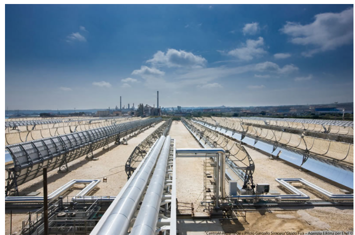
Figure 7. Enel's Archimede Concentrating Solar Plant stores thermal energy for use at a natural gas-fired combined-cycle plant on site, enhancing plant flexibility.
