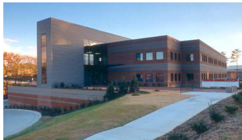
Advanced Energy's office on North Carolina State University's Centennial Campus in Raleigh, NC
